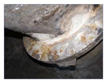
Figure 2. The reducer prior to repair.
